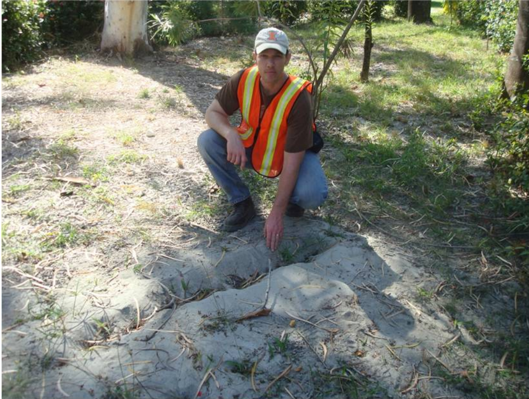
Figure 7.13. Sand blow and ejecta formed at coastal failure site near village of Fouche. Approximate image coordinates: 18^{\circ}25'35.08''\text{N} , 72^{\circ}43'31.70''\text{W} .
