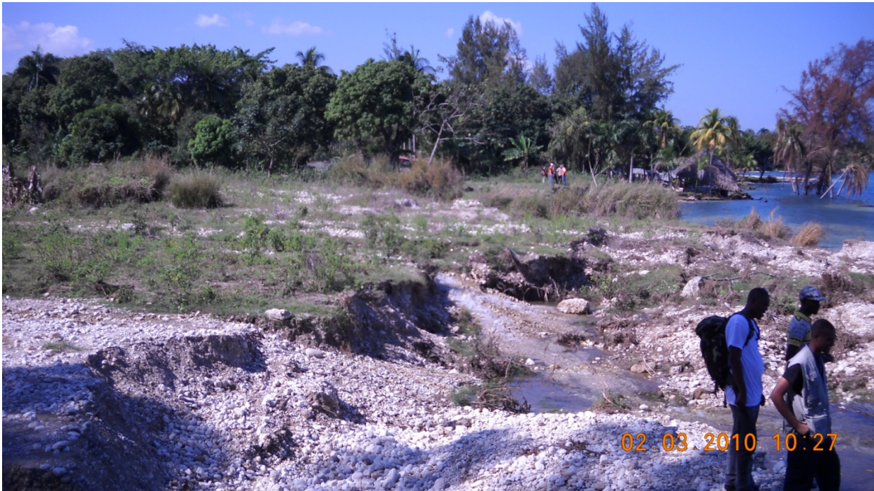
Figure 7.10. Scarp of coastal landslide near village of Fouche. ( 18^{\circ}25'34.01''\text{N} , 72^{\circ}43'34.60''\text{W} looking westward).
