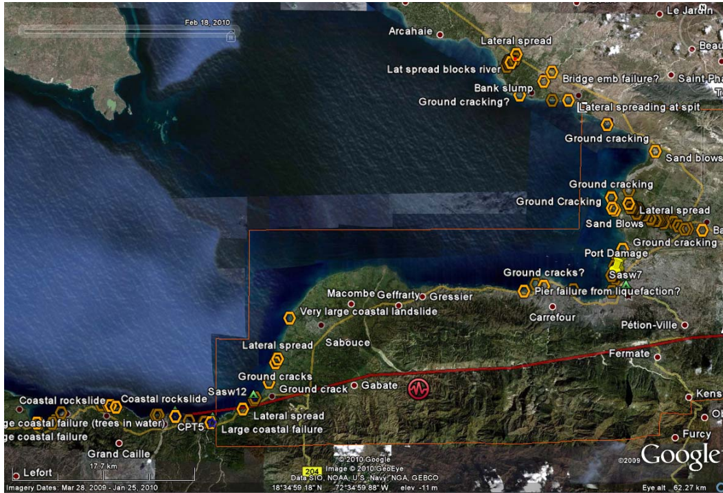
Figure 7.1. Potential liquefaction, lateral spreading, and coastal failure sites identified from post-earthquake aerial photography (sites identified as open hexagons). Imagery courtesy of Google Earth.
