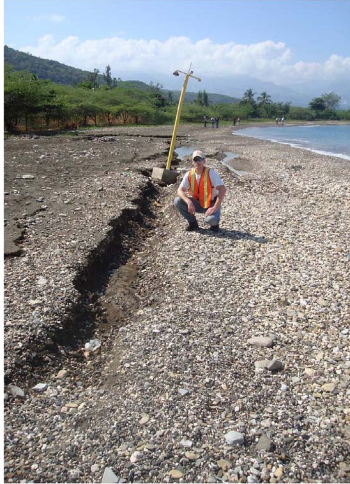
Figure 7.4. Cracking and lateral spread along coastline near village of L'Acul. ( 18^{\circ}26'48.81''\text{N} , 72^{\circ}41'11.92''\text{W} looking west).
